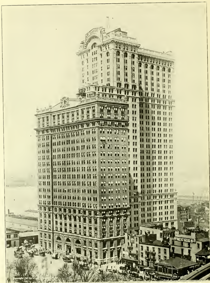
THE WHITEHALL BUILDING—Located on Battery Place, between West and Washington Streets, is the largest, single office building in the world. The original building, 20 stories, 254 feet high, was finished in 1903 at a cost of $1,000,000, the new addition of 32 stories, 416 feet high, was finished in 1911 and cost $4,600,000. The building covers 21 city lots.
